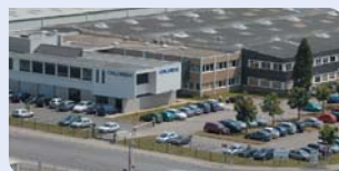
Lyon, France Industrial UPS manufacturing R&D centre
