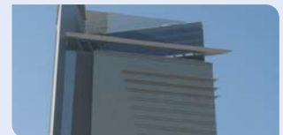
Dubai, UAE Middle East HQ
